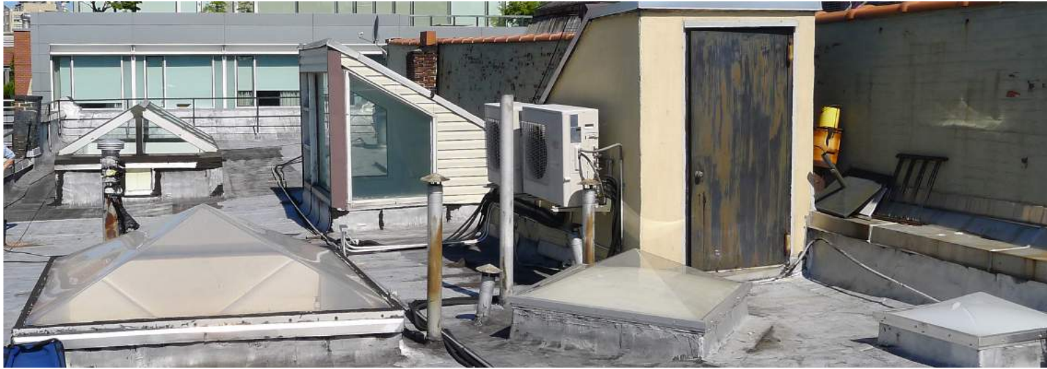
ROOF LOOKING SOUTH
